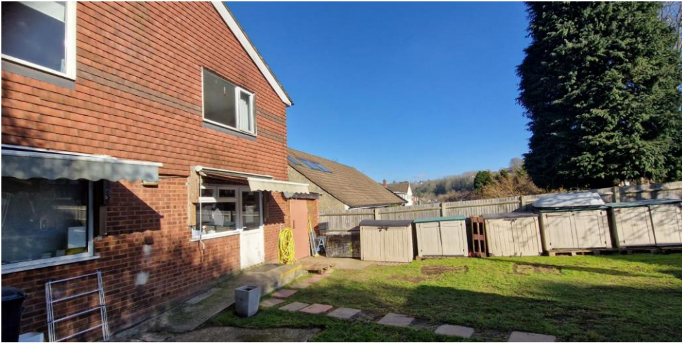
Figure 9: Photo showing view to No.121
